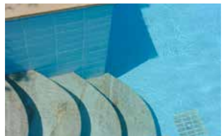
EASY STEP ACCESS TO POOL Safe and secure access to the pool
